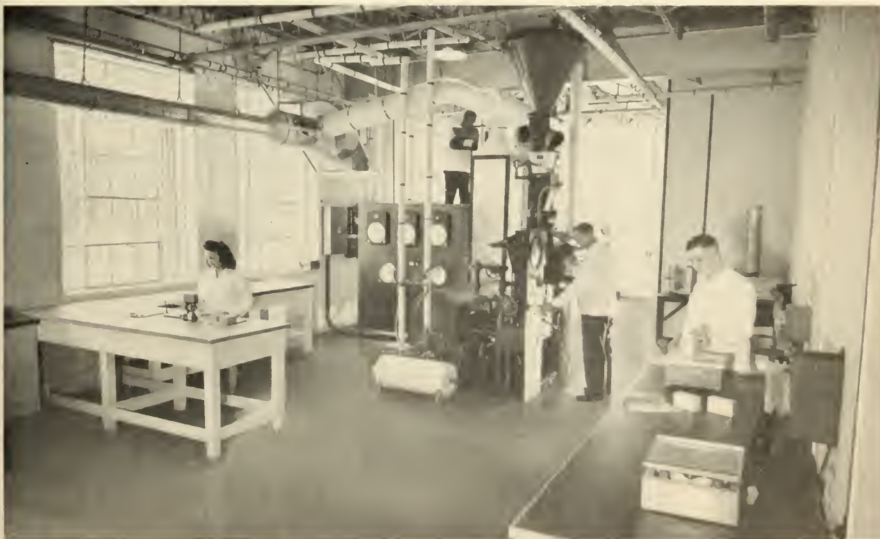
FIGURE 8.—Interior of the food-compression laboratory at the Agricultural Research Center at Beltsville, Md., showing the special 40-ton hydraulic food press developed for the work, with the instrument panel and conditioning bins in the background. Food blocks are being weighed and wrapped at the work tables.
